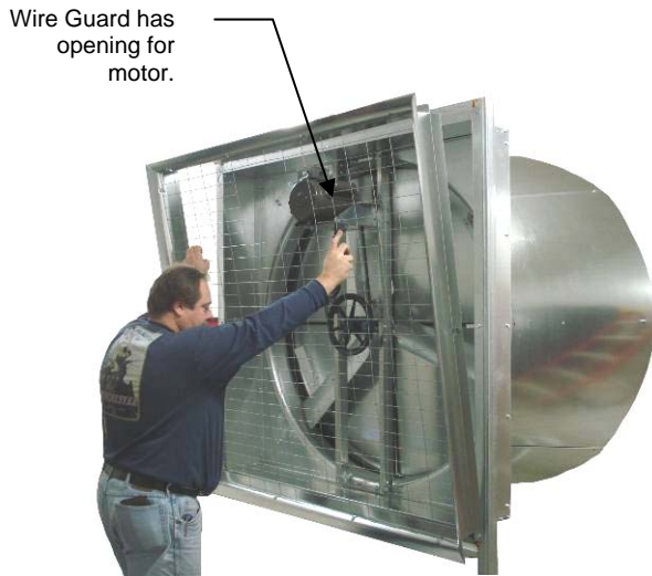
Figure 14: Install Fan Inlet Frame
